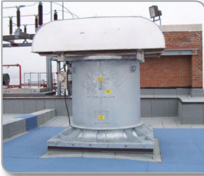
MODEL VJ DIRECT DRIVE VANEAXIAL FAN
